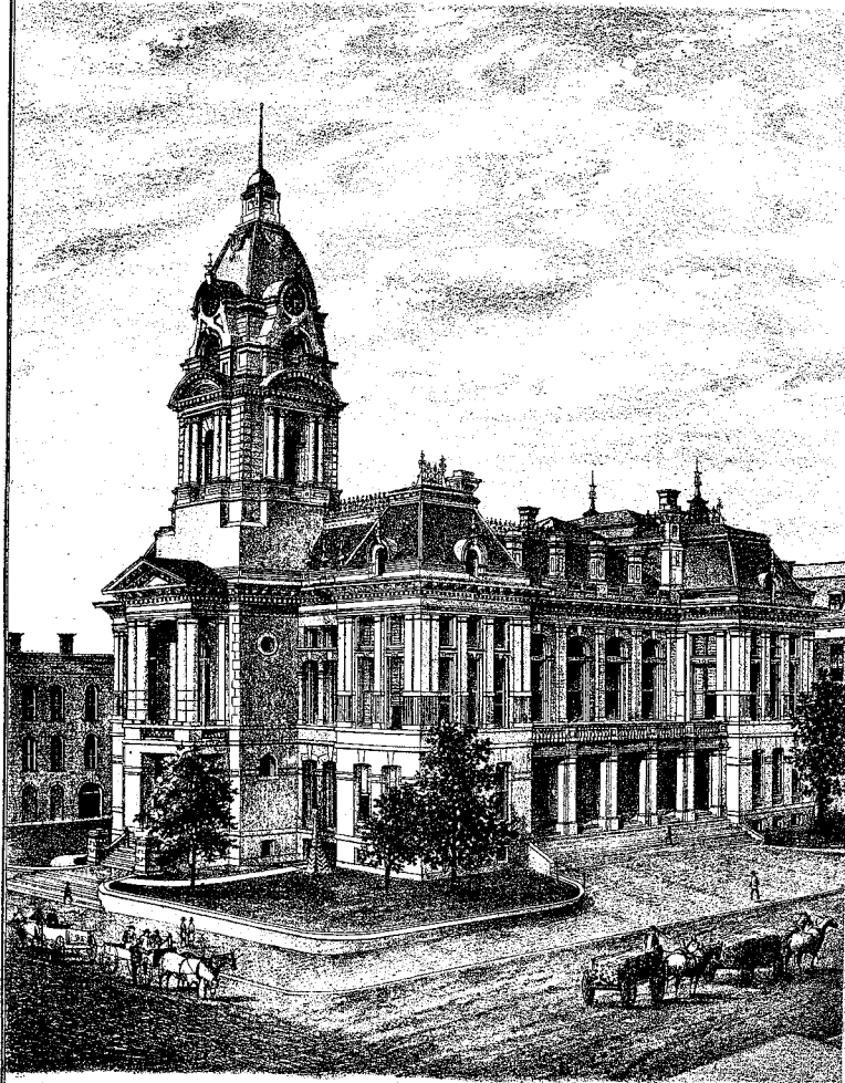
MONTGOMERY COUNTY COURT HOUSE
